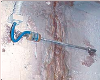
• Model 4420 Crackmeter installation.
